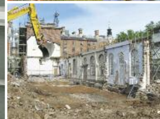
Stripping the building back to its core.
