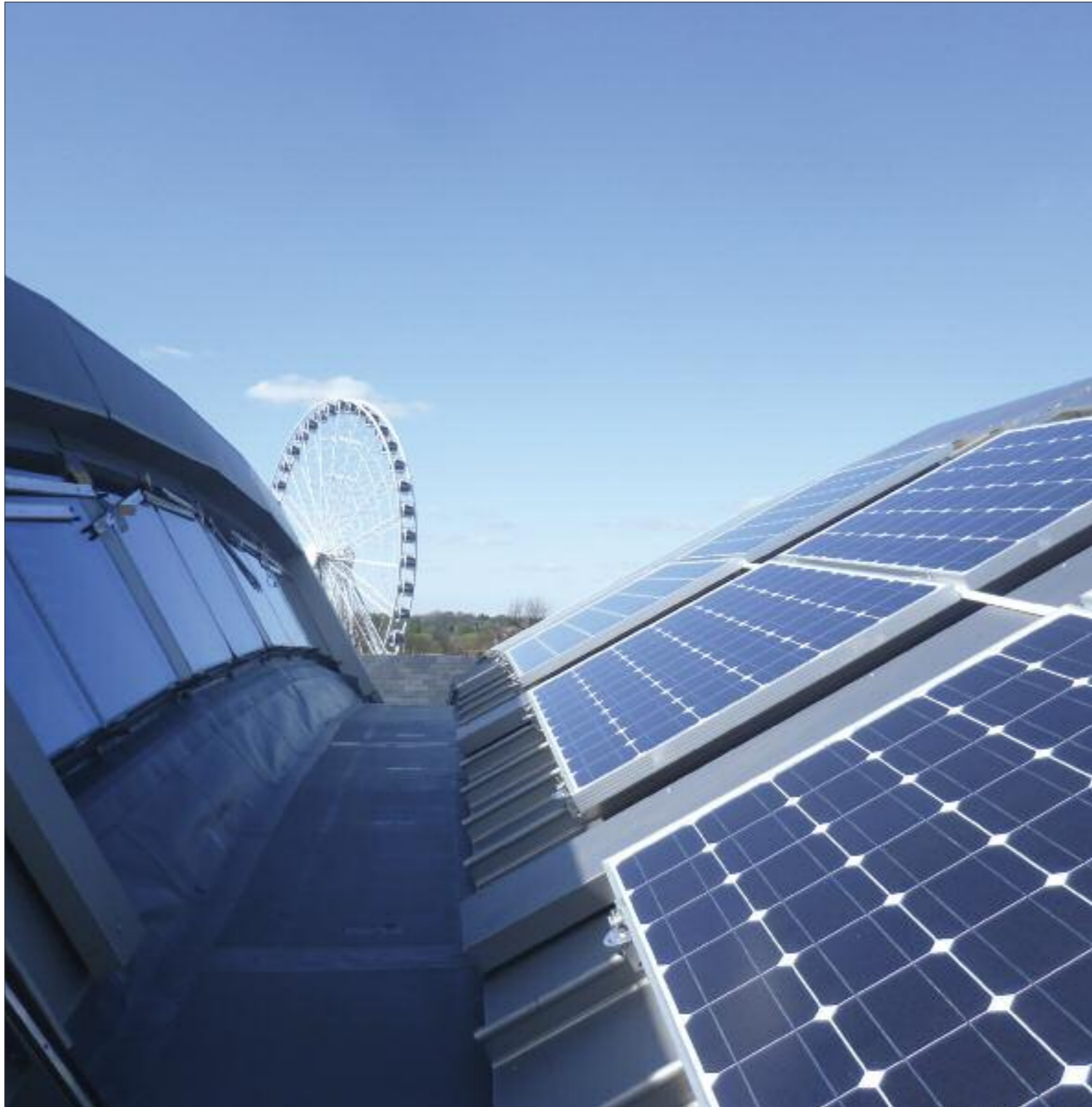
The north light roof features solar PV panels on the south facing planes. The basement houses biomass boilers and CHP units.
